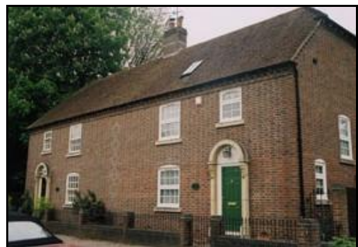
Photo 37: New development next to George House, East Street
