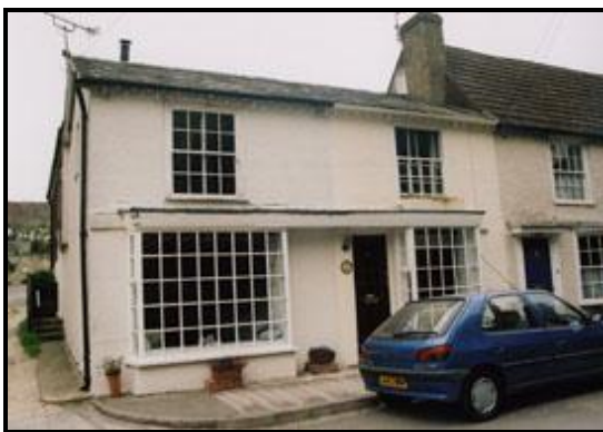
Photo 28: Nos. 6a and 6b High Street
