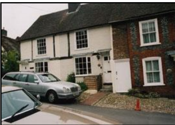
Photo 20: Hilltop and Hillside, High Street
