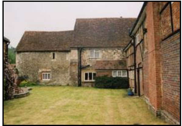
Photo 18: Rear wing of Manor Farm House
